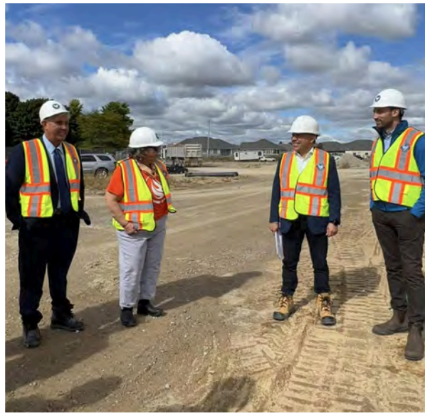
Anthony and Stephen Lecce at the construction site for a new Kingsville School
